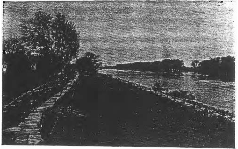
Levee Maintenance • North Pocket Area
